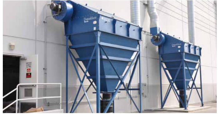
CPC-24 - Paper tissue manufacturing 7,600 cfm (12,910 m 3 /h)
